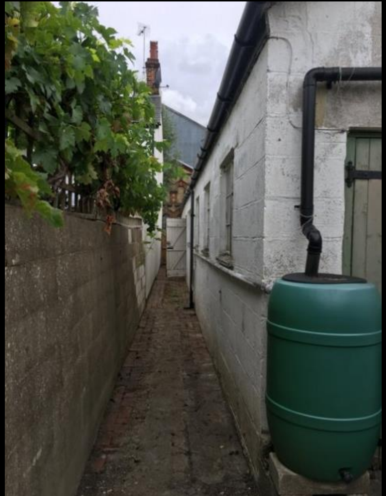
Side and rear elevation of the existing building
