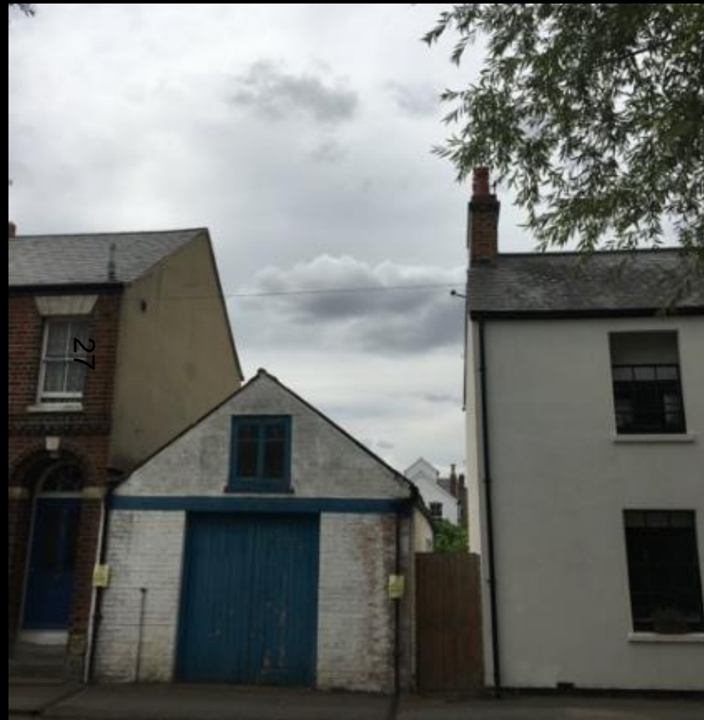
View of the existing front elevation
