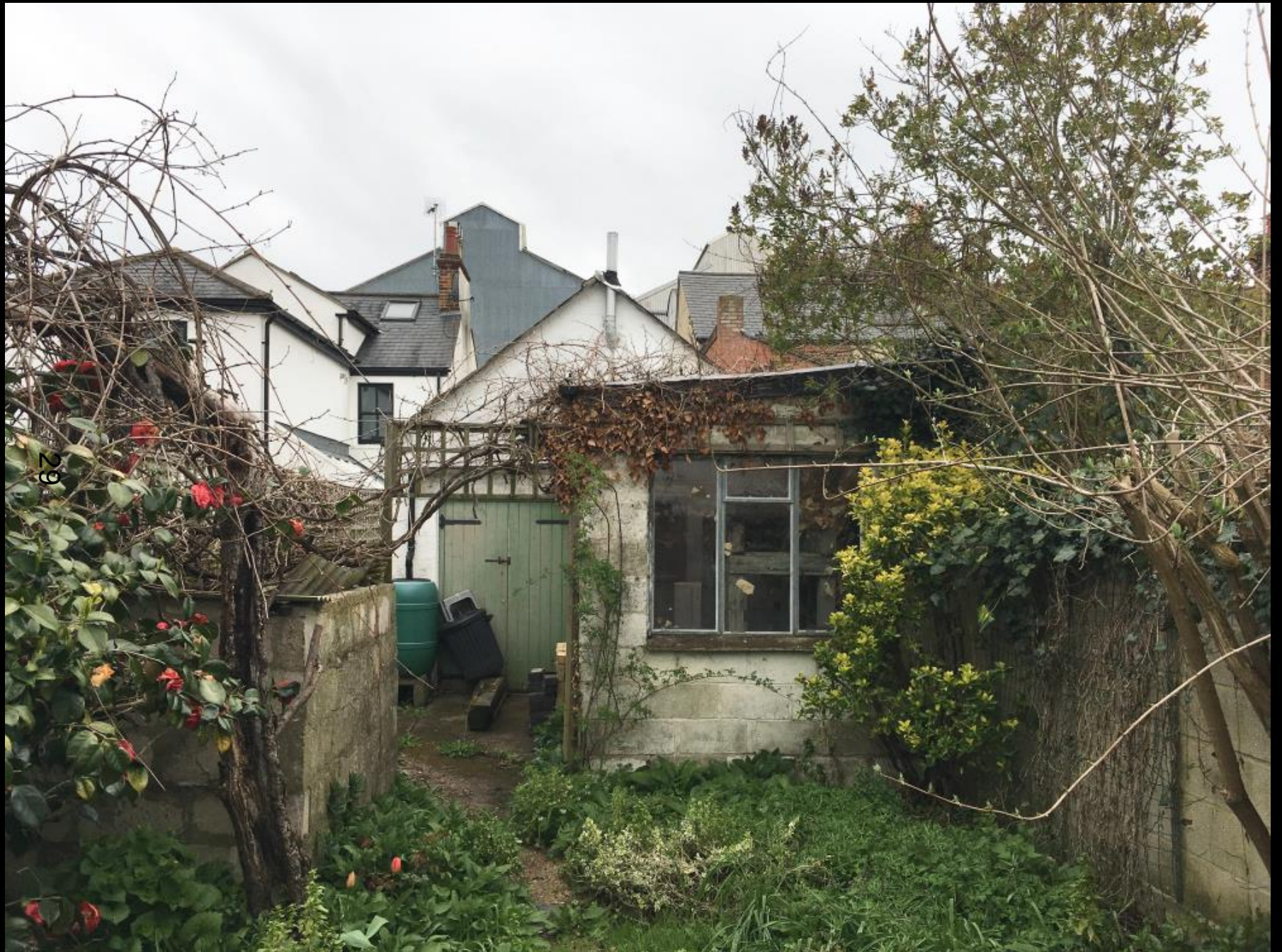
View of the existing rear elevation
